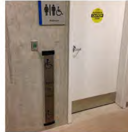
Figure 8: Elongated power-operated door control usable at multiple heights
