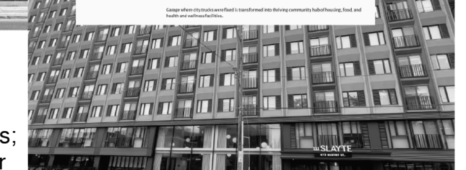
Converting office space to apartments in Ottawa
